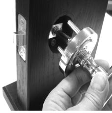
\$\insert 5\$) Insert the remaining lock-half into the public (outside) side of the door. Note that the two threaded mounts on this lock-half insert into the larger tubes on the other lock-half.
