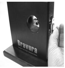
⊕ 2a) Insert latch mechanism into door. If using a <u>privacy</u> latch, make certain the threaded button is facing the side of the door from which you wish to lock the door
